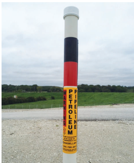
Our pipeline markers can be typically identified by the black and red bands at the top.
